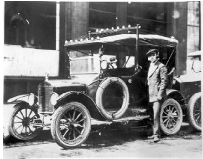
Antennas can be a problem
