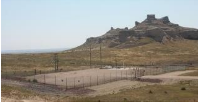
Typical Minuteman Launch Facility
