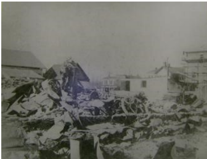
Devastation from the 1905 fire in Manassas
