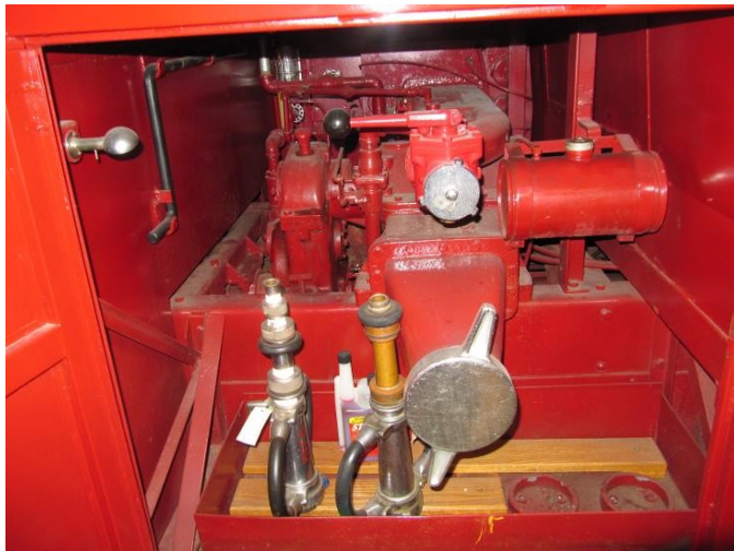
Right side view of pump compartment
